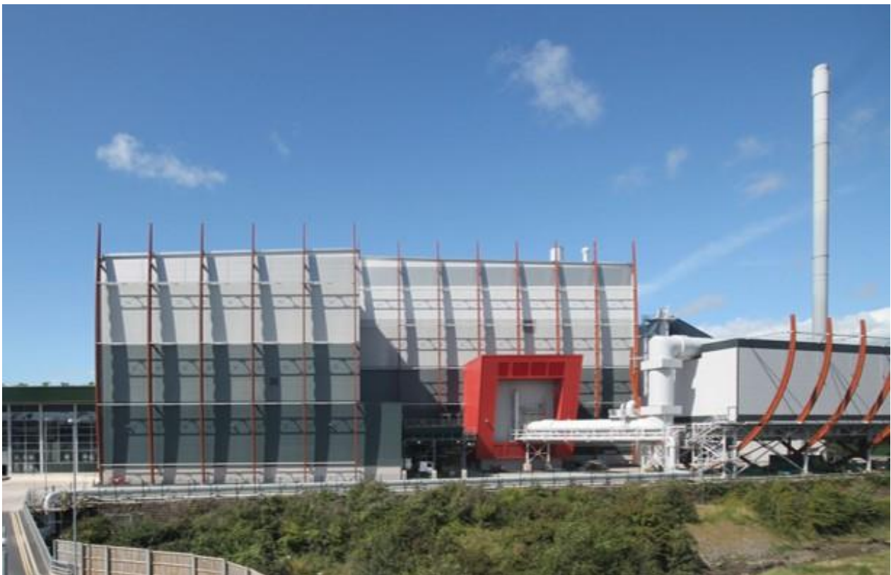
Plate 5-3 Indicative Image of a Combustion Plant
